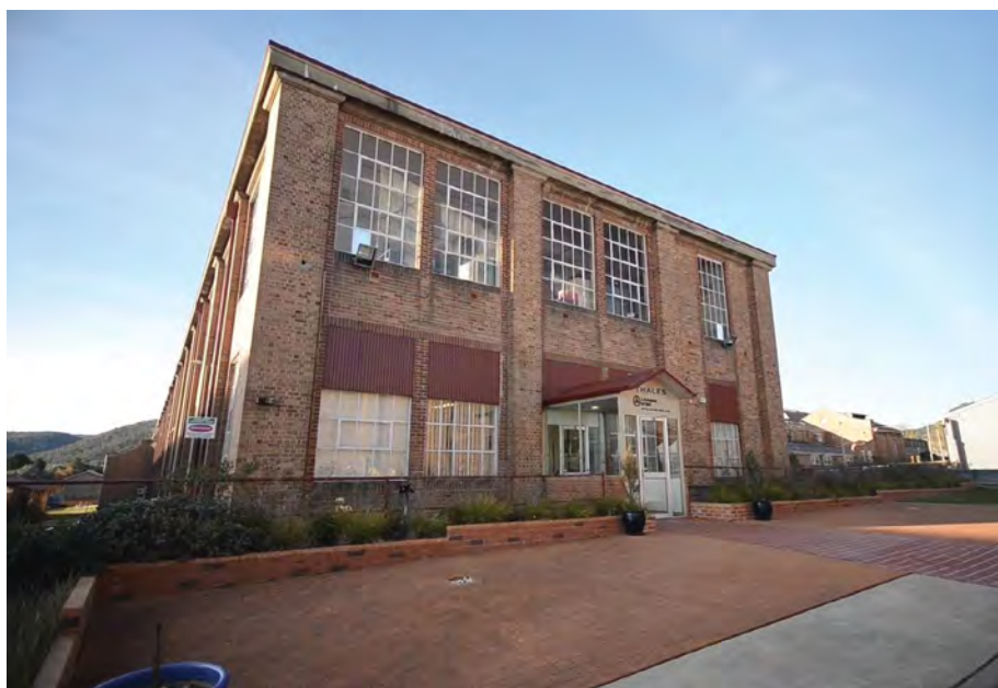
Building 52, the main office and manufacturing building in Lithgow today. Image courtesy ThalesGroup Australia.
